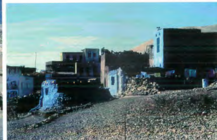
Village de Gournah...avant destruction.
